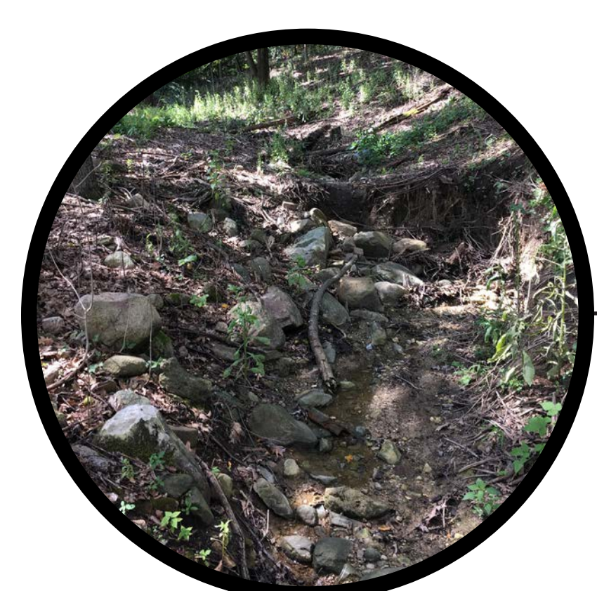
Removal of an earthen dam and water control structures will restore highly eroded ravine complexes.
